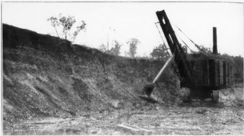
Steam Shovel in Pit.
